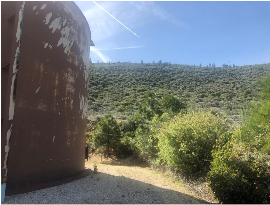
The 2:1 slopes behind the existing water tank populated with mature vegetation
